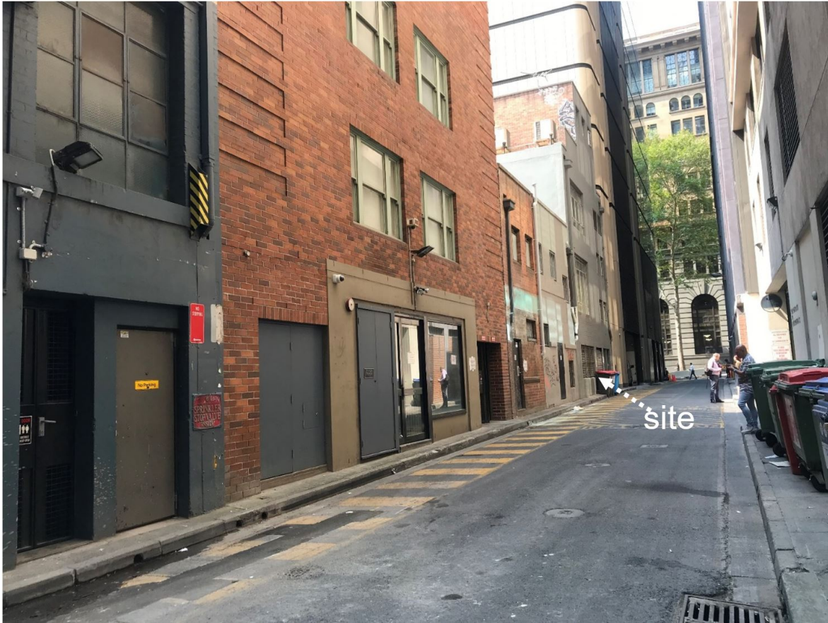
Wynyard Lane looking south
