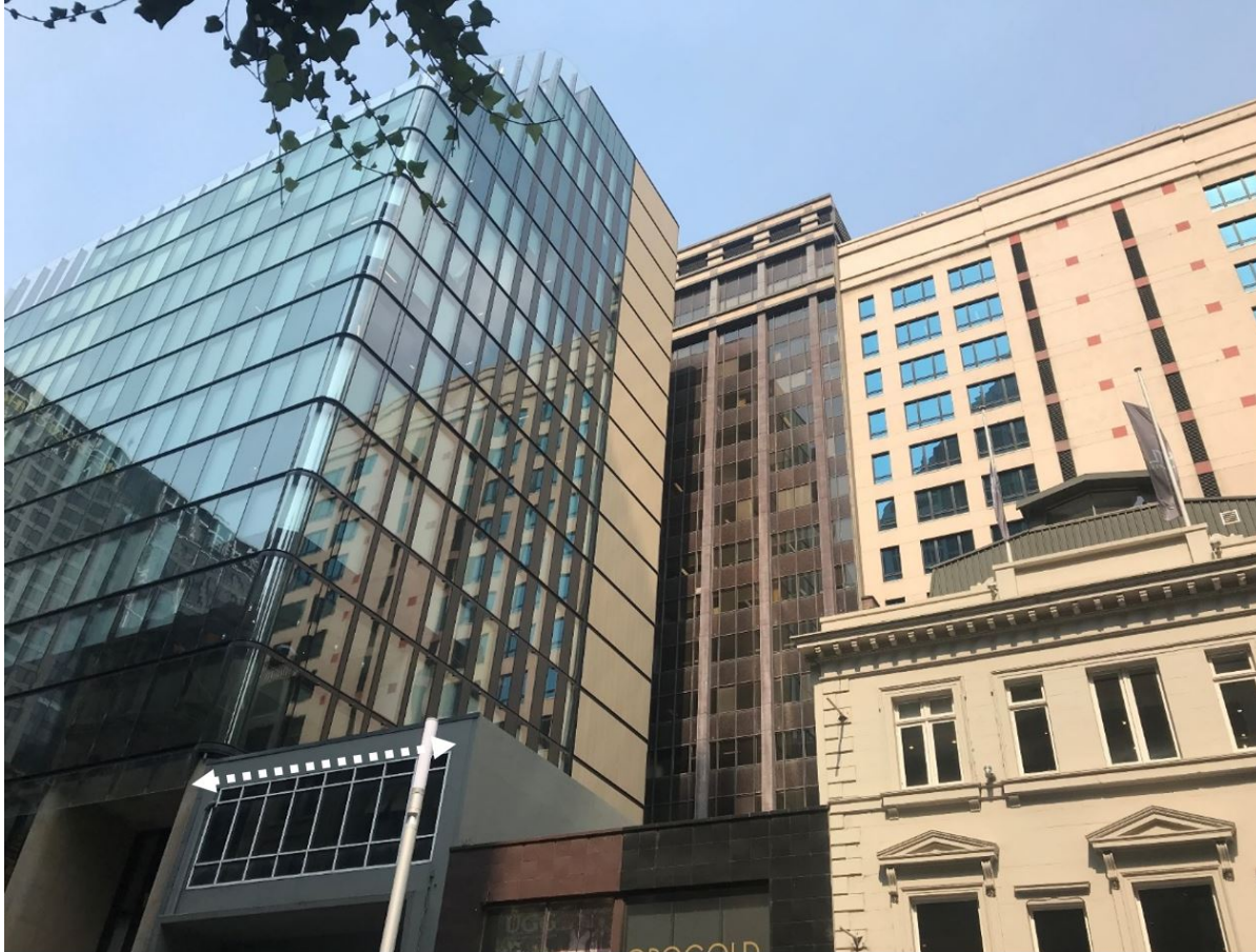
333 George Street adjacent to site
